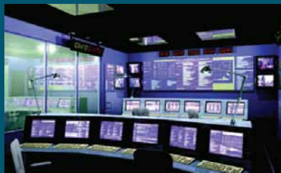
Air Traffic Control System
